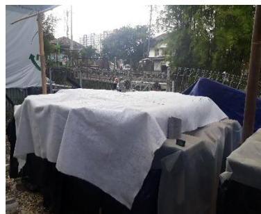
Gambar 34. Rawatan keras metode wet geotextile non woven
