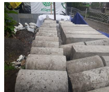
Gambar 35. Rawatan keras metode curing compound
